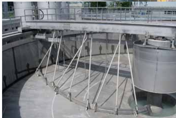
Separation by solid circular clarifiers.
